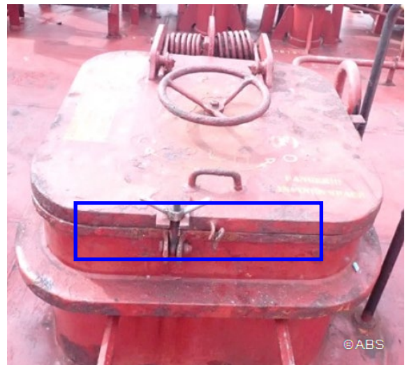
Faulty closing mechanism and dogs of bobby hatch cover restrict the wheel to positively close
