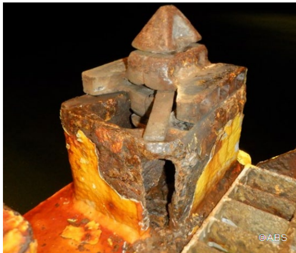
Twist lock foundation at container housing cracked
