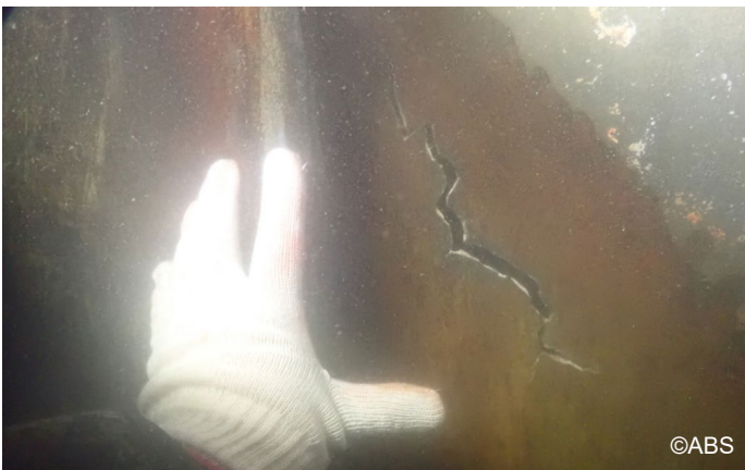
Owners are to report all damages that may affect classification. Side shell found damaged outside - before
