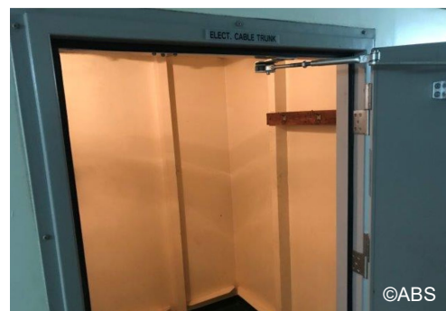
Self-closing fire door after repair
