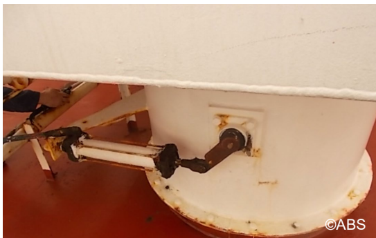
Fire damper linkage repaired
