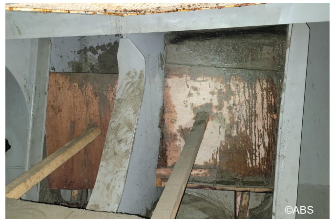
Side shell plating with cement box – temporary repair
