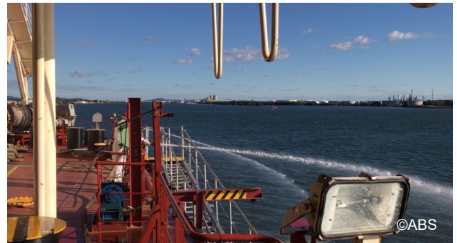
Emergency fire pump testing after repair to defective controller
