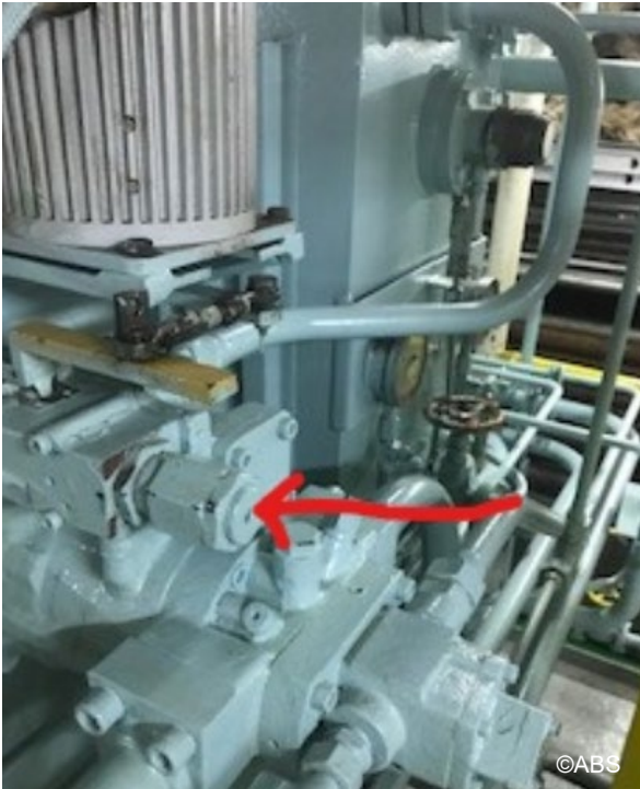
Steering gear repaired for rudder centering adjustment bolt
